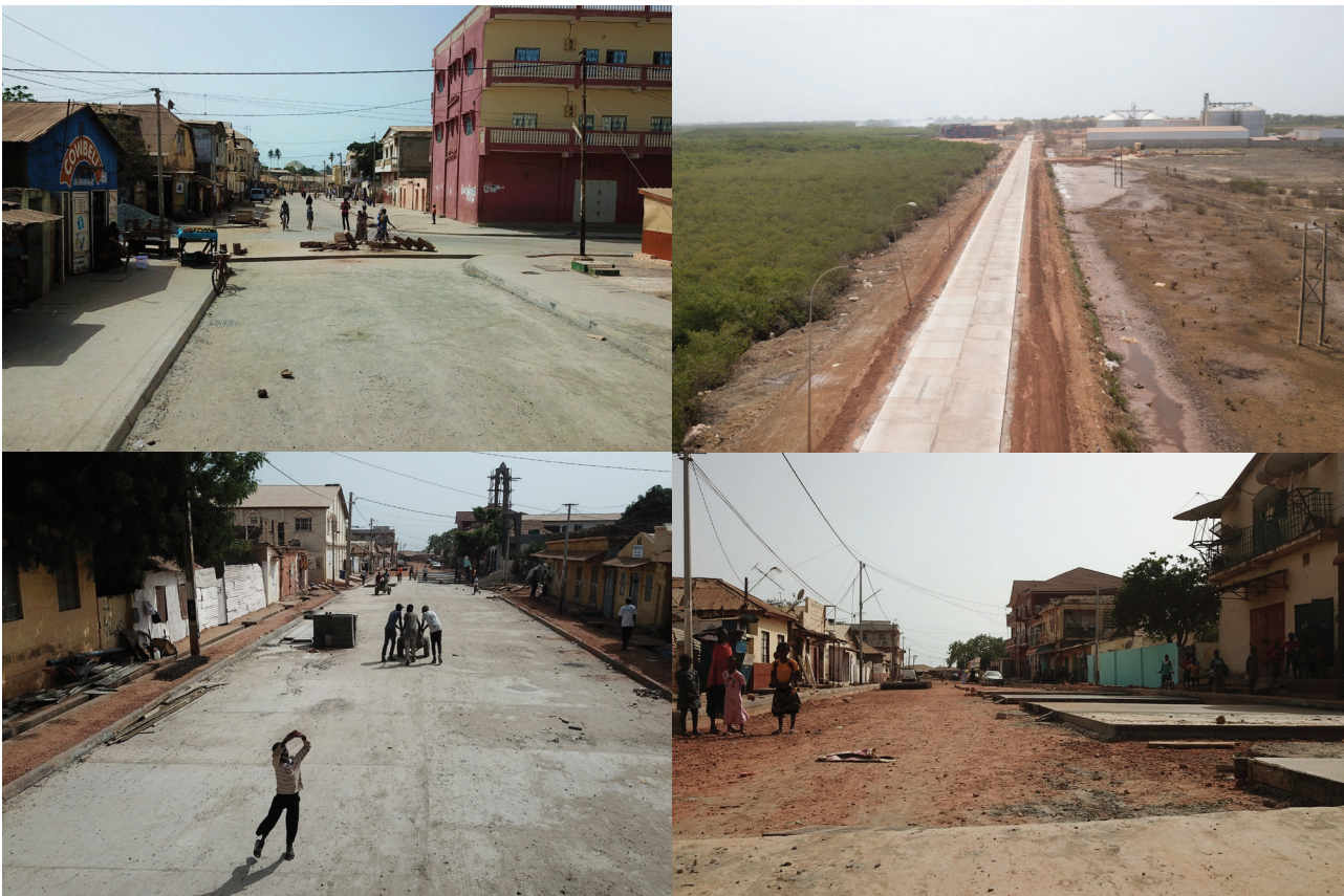
Construction work on the Banjul Rehabilitation Project
