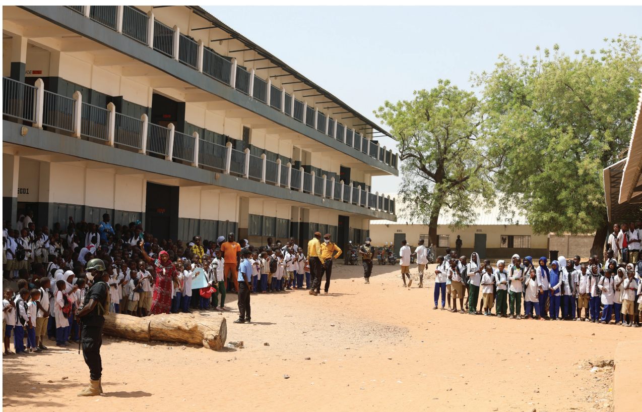
New Classroom Block constructed to expand Koba Kunda Lower Basic into a Senior Secondary School
