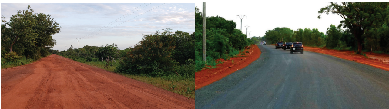
Hakalang Road during Construction
