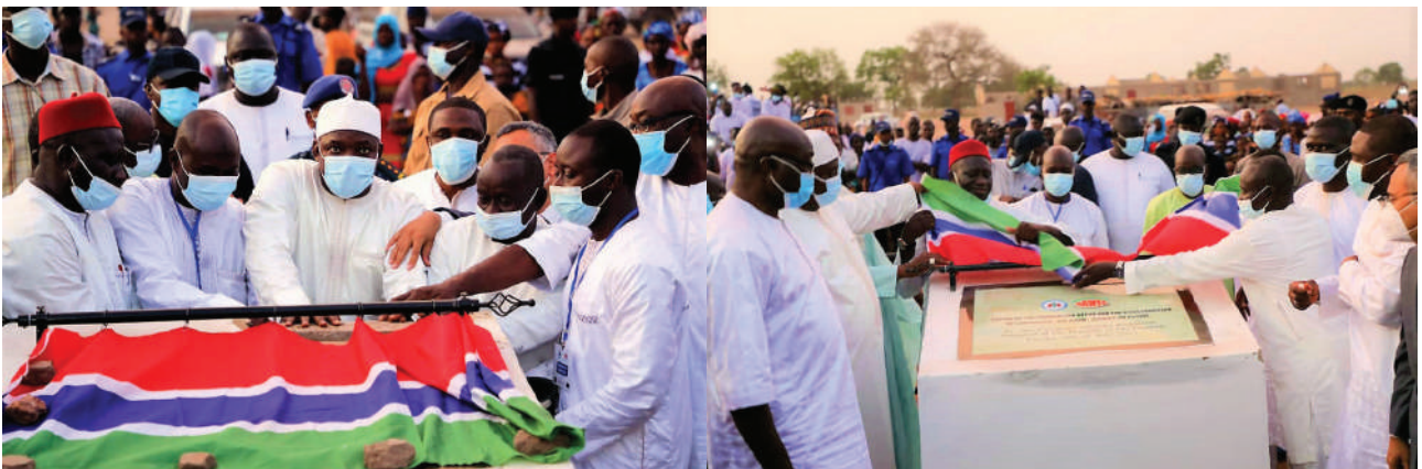
LAYING THE FOUNDATION FOR THE 30KV LAMINKOTO-DIABUGU BATAPA ELECTRICITY LINE
